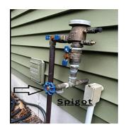
**IMPORTANT** – Before you start your system in the spring – put the plug back in place on the backflow and/or close the spigot to prevent water gushing when the system is activated. Turn the water on **SLOWLY!**
